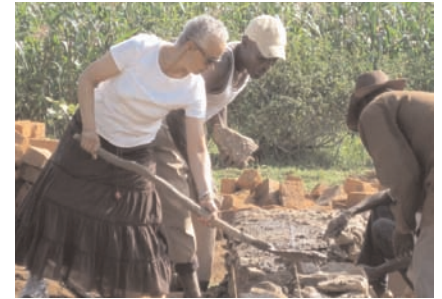
Joan working on the foundation
